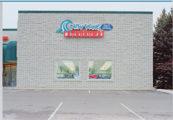
The 3,500-square-foot laundry features ample parking and a paging system to alert customers when their wash is finished.
